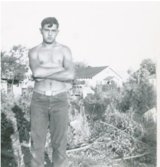
Georgie at 746 South Chelan Street.
