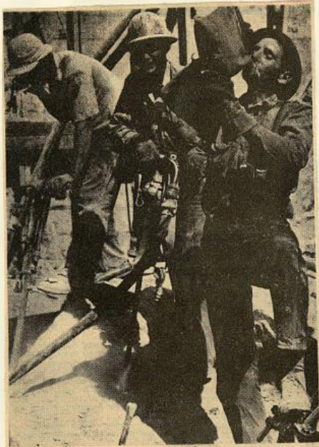
ROCK MEN AT GRAND COULEE —Nearly 4500 men find employment in the construction of Grand Coulee dam on the Columbia river in Washington. This jackhammer crew is at work smoothing the bedrock to receive concrete. A concrete form is in the background. Time out does double duty as he takes a drink without interrupting his smoke.
