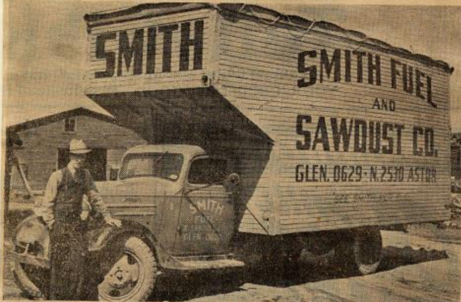
This huge conveyance is being used by the Smith Fuel and Sawdust company to rush shavings to Coulee dam to aid in plugging the leak in the coffer dam and save the giant structure when the rush of spring water begins. It carries 10 cords of shavings at a time and is making two trips daily in addition to another four-cord truck making two daily trips. Corliss Smith, proprietor of the company, is shown with the truck.
