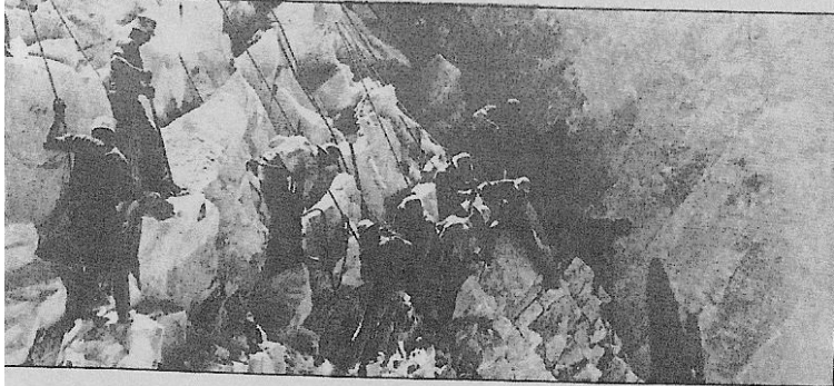
WORKERS HAD TO USE ROPES FOR SECURITY WHILE SHAPING BEDROCK WHICH SUPPORTED THE FOUNDATION
