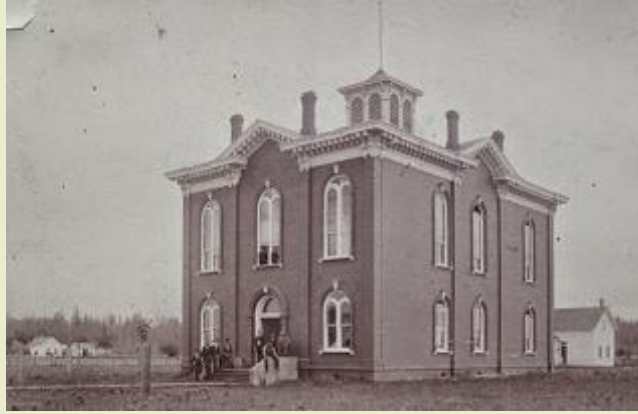
32. Washington County Courthouse in Hillsboro, built in 1873, 1st & Main The newer jailhouse built in 1870 is to the right Richard Wiley's home is on the left
